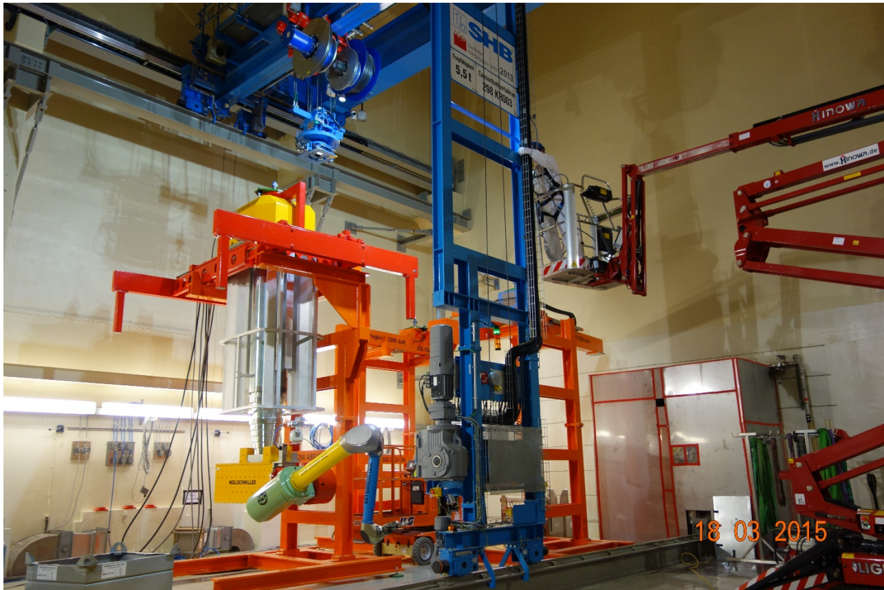
Fig. 2: Electrical Master Slave Manipulator (EMSM) with Telescope and auxiliary crane system
